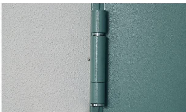
Hinge with self-closing spring.
